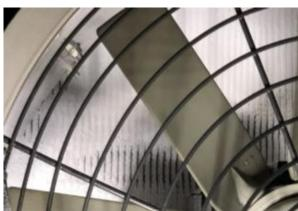
Air outlet side on the same evaporator covered blocked with ice
